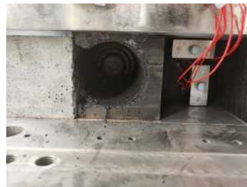
(a) 钻孔卸压
